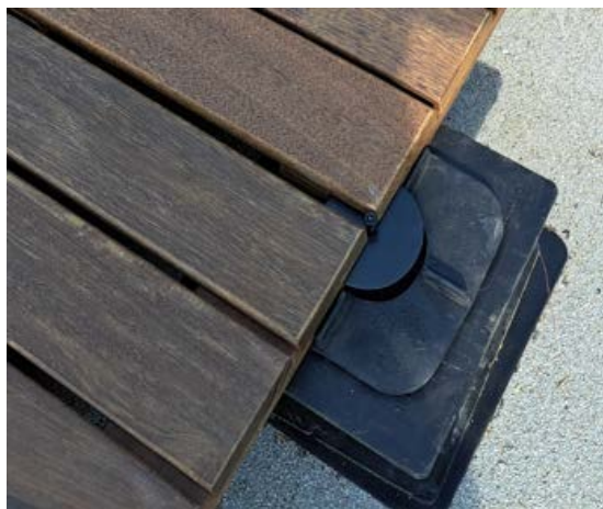
IPE with Lok-Down Hardware and Terra Stand
